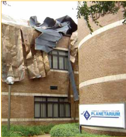
Hurricane damage at Seminole Community College
